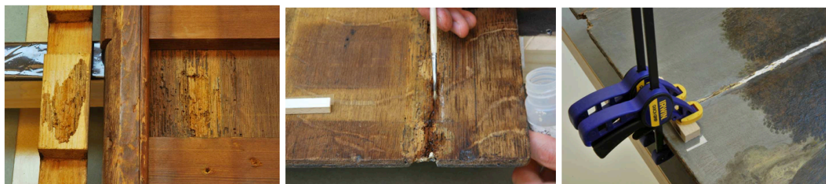
Fig. 3 The insect damages and the restoration. The movements of the boards.
